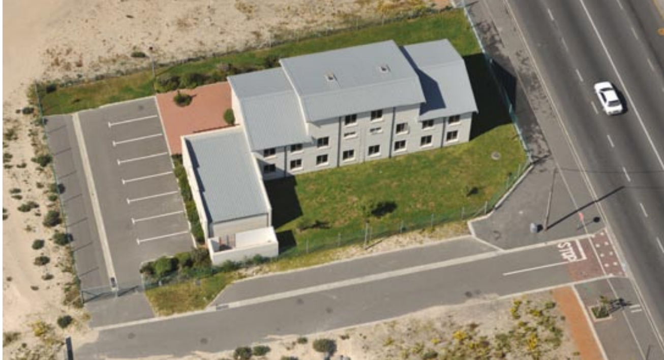
Aerial view of Show Village
